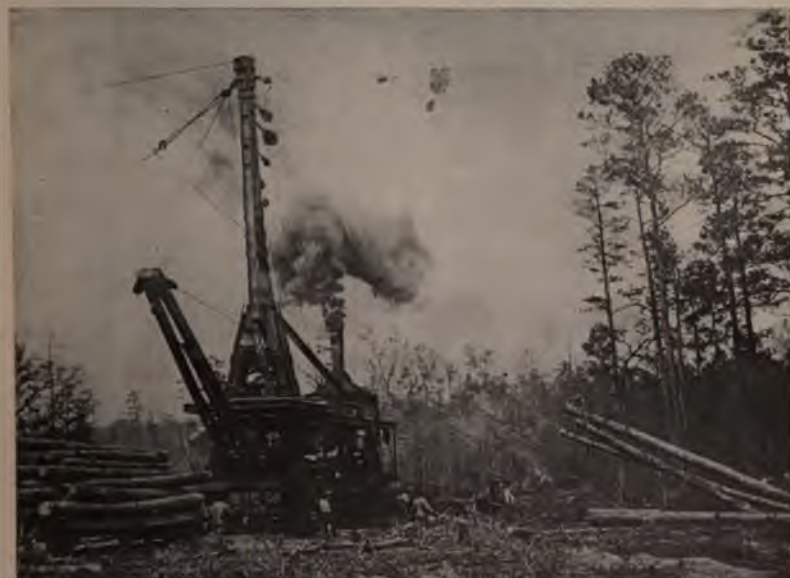
FIG. 52. — A Steel Spar Cableway Skidder showing Loading Boom in Front.
